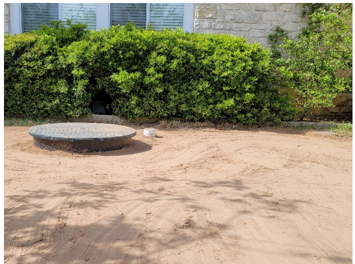
Examples of post-construction ground covering and exposed grinder pump tank completed during LMUD install.
