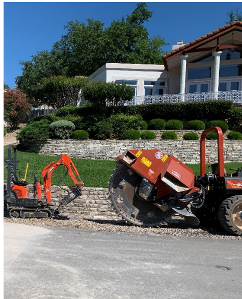
Trenching for main line and service line | Examples of equipment that may be used | Installing service line to grinder pump tank
