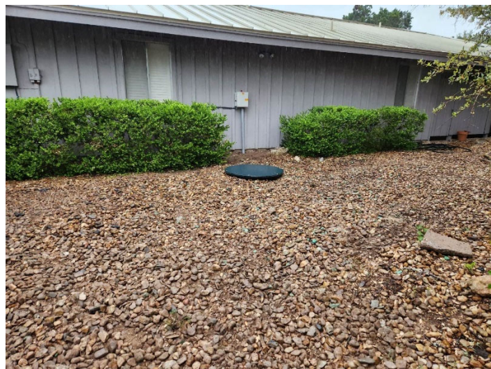
Examples of grinder pump tank and control panel ground covering completed by customers
