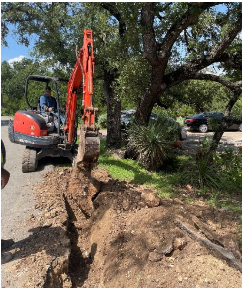
Trenching for main line and service line | Examples of equipment that may be used | Installing service line to grinder pump tank
