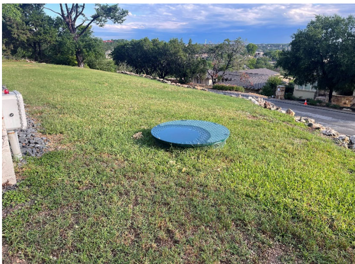
Examples of grinder pump tank and control panel ground covering completed by customers
