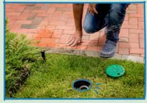
As you get ready for warmer weather, make sure you connect hoses and pipes in your irrigation system well to avoid leaks.
